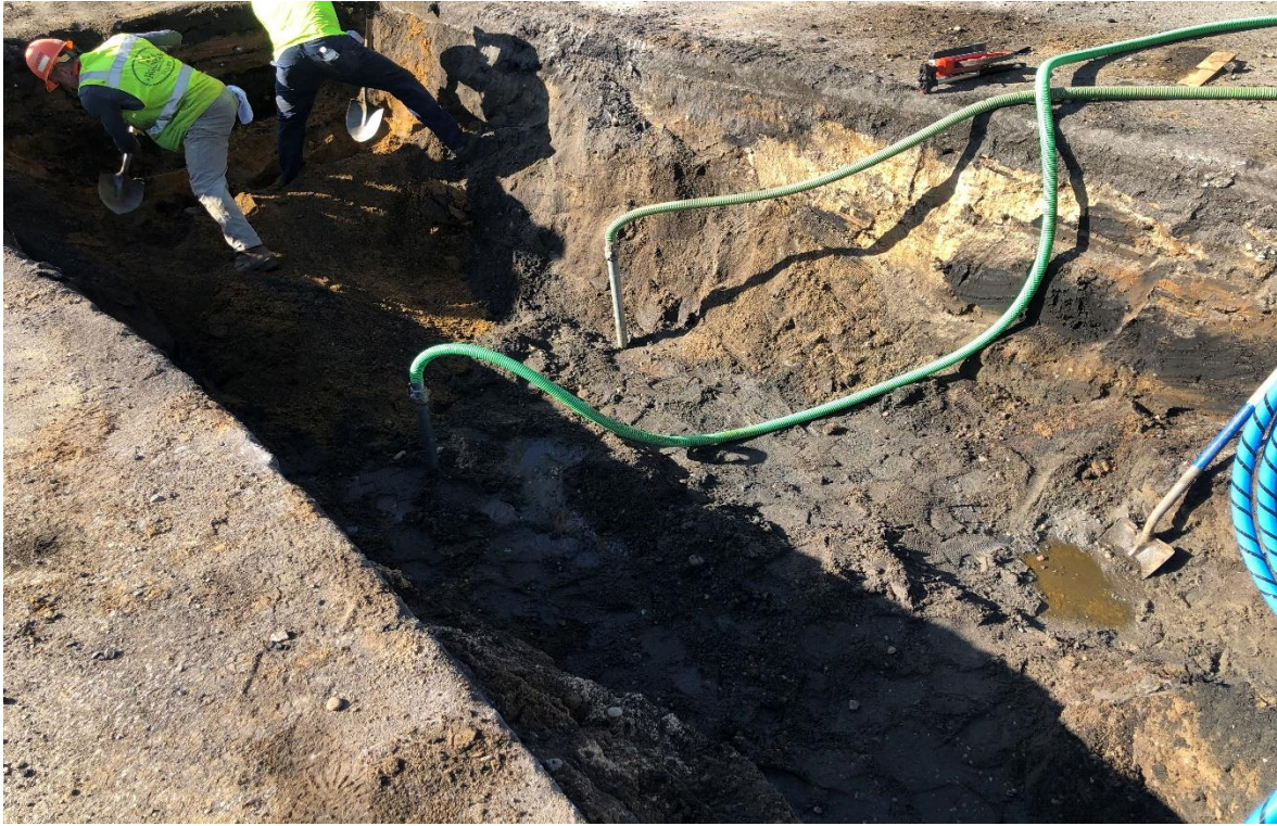
Photo 3: Trench and dewatering points in ROW.
