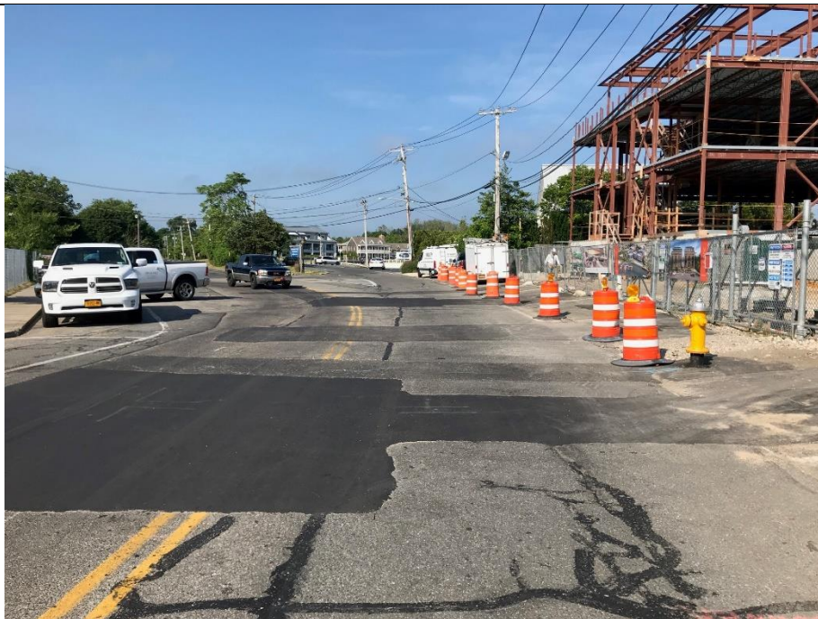
Photo 4 – Repairs to asphalt following 2 West Water Street utility connection project on Long Island Avenue, looking west.
