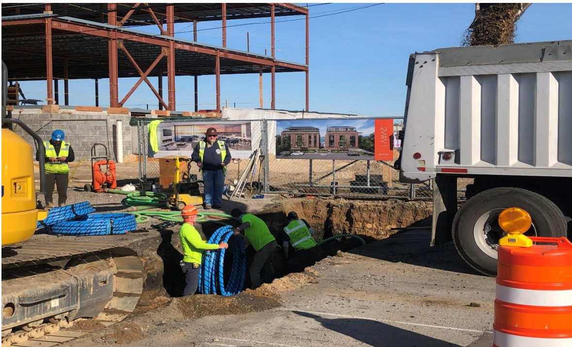
Photo 4: View of water service line installation in ROW.
